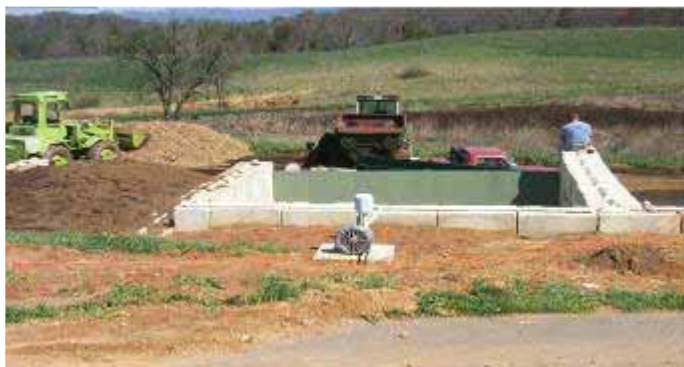
Gambar 9. Aerated compost bins
